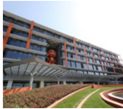
Photo courtesy of Alibaba Group
